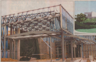
The company can supply and fix walls, posts, flooring systems, trusses and other framing components
